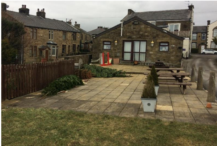
View north towards the dining room extension
