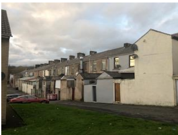
Rear Elevations of the terrace block the property is part of.
